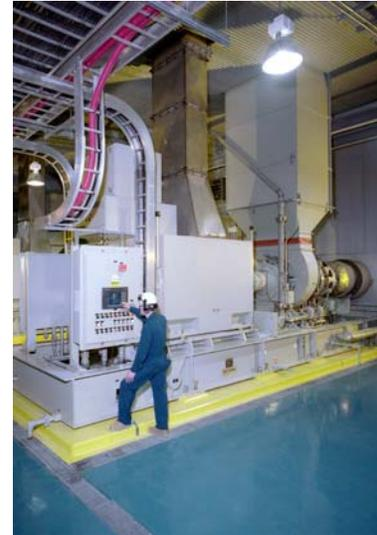
*A leading industrial manufacturing plant in Deer Park, Texas, commissioned four gas turbine generator sets to provide 18MW of reliable heat and power to support the company's operations and to protect against power outages.*
